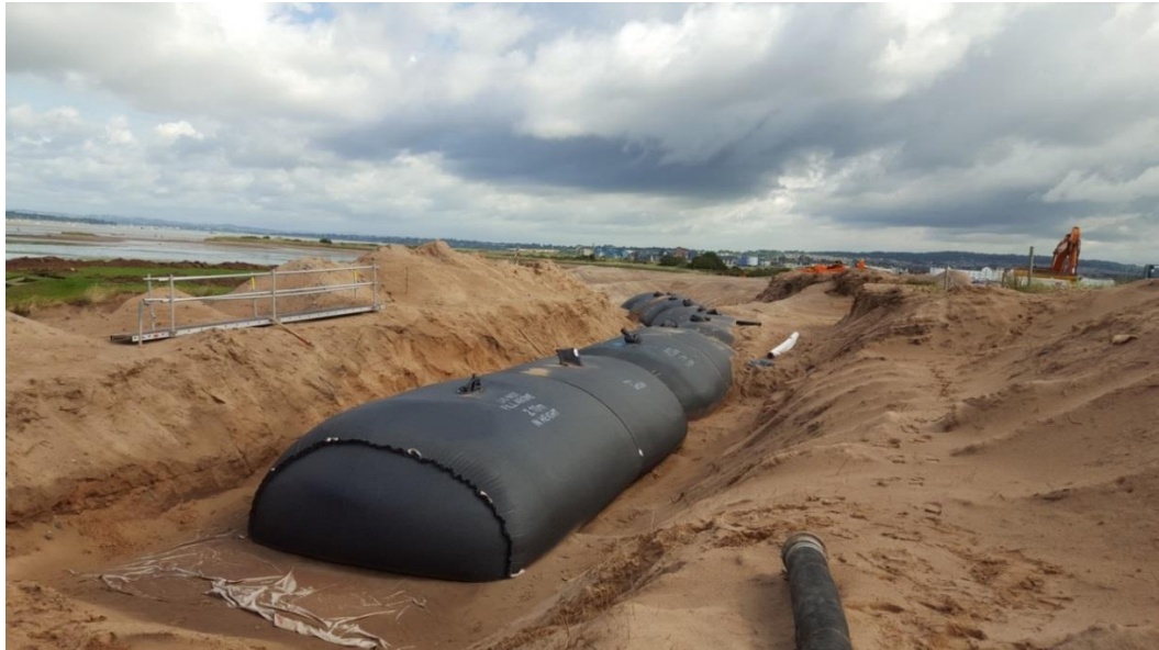
Geotube instalation at the neck, Dawlish Warren, 23 rd July 2017, Lee Collins
